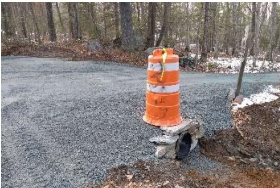
Newly raised roadbed and new culvert at Erie and Birch
